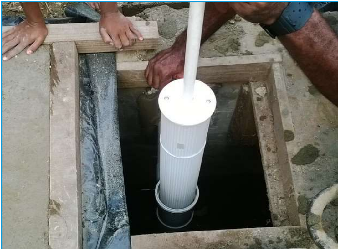
Figure 5 Septic Tank filter being inserted into an outlet tee.
