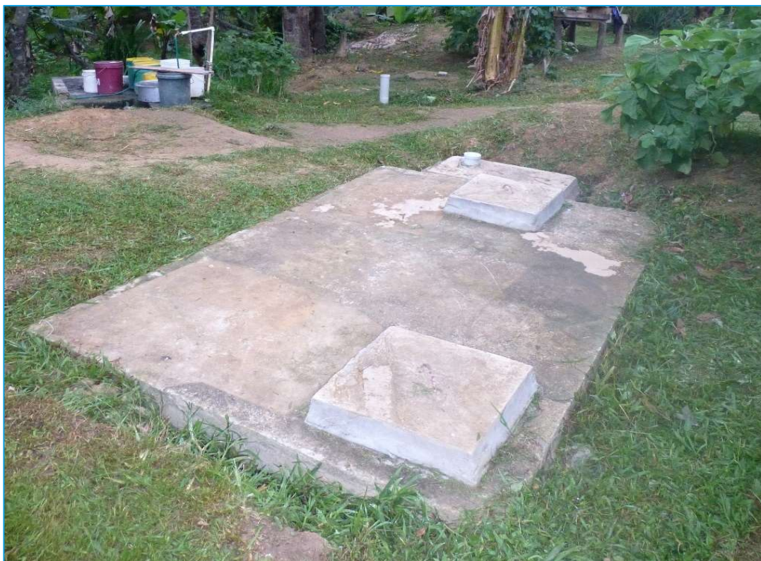
Figure 7: Completed household blackwater septic tank for 6-8 people. Dosing chamber and land application system vents are visible on far side of tank.
