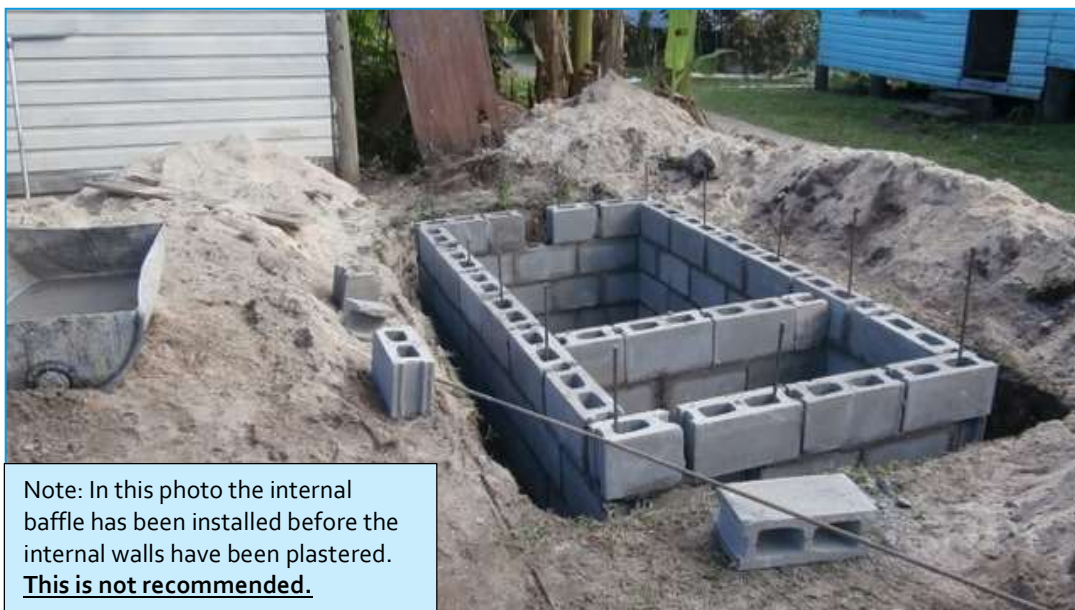
Figure 4: Septic tank under construction.
