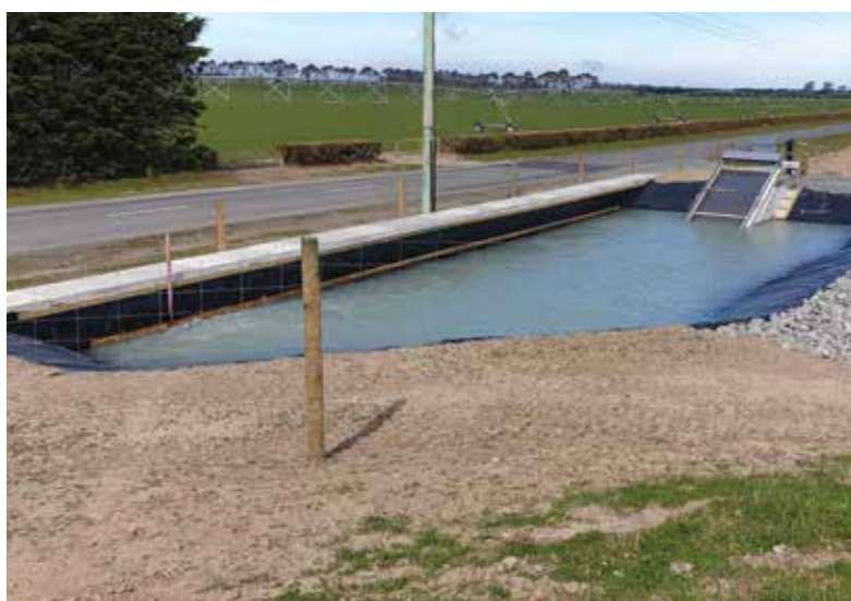
The pipe intake on the Acton Irrigation Scheme. Water from the small pond then runs through a filter and into the piped delivery system. [Rod Mckay]
