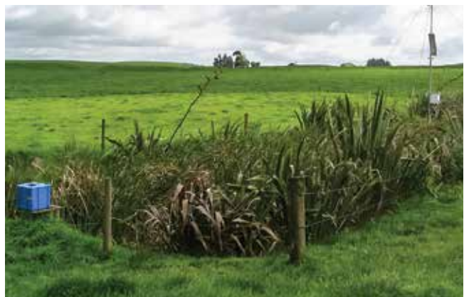
Constructed wetlands intercept and treat tile drainage flows from grazed pasture to natural waterways. (Chris Tanner)
