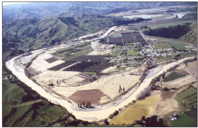
Figure 10. Damage caused by ex-Tropical Cyclone Bola.
