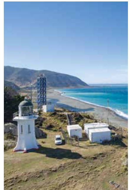
NIWA's Clean Air Monitoring Station at Baring Head in Wellington. (Dave Allen)
