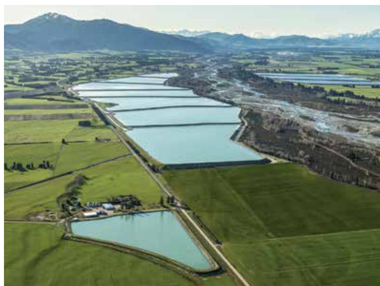
Rangitata South Irrigation Scheme. (Rooney Earthmoving Ltd)
