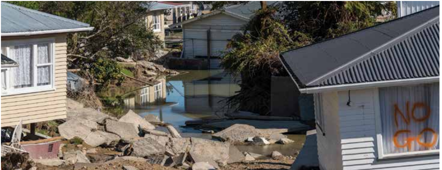
Houses damaged in the 2017 Edgcumbe floods after Cyclone Debbie swept through the Bay of Plenty. (Dave Allen)
