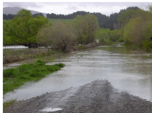
Flood water on Waiotaka Rd.
