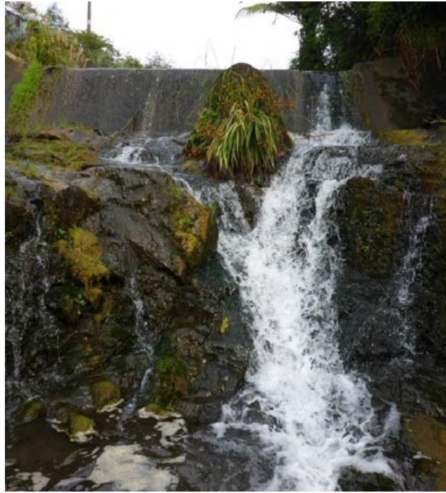
Figure 6-9: A weir built on top of a natural waterfall in Waitawhara Stream, Waikato. Although not designed as a selective barrier, the weir and waterfall prevent koi carp, goldfish, perch, rudd, gambusia and catfish from accessing headwater habitats whilst allowing the passage of banded and giant kōkopu and shortfin and longfin eels. Credit: Cindy Baker.
