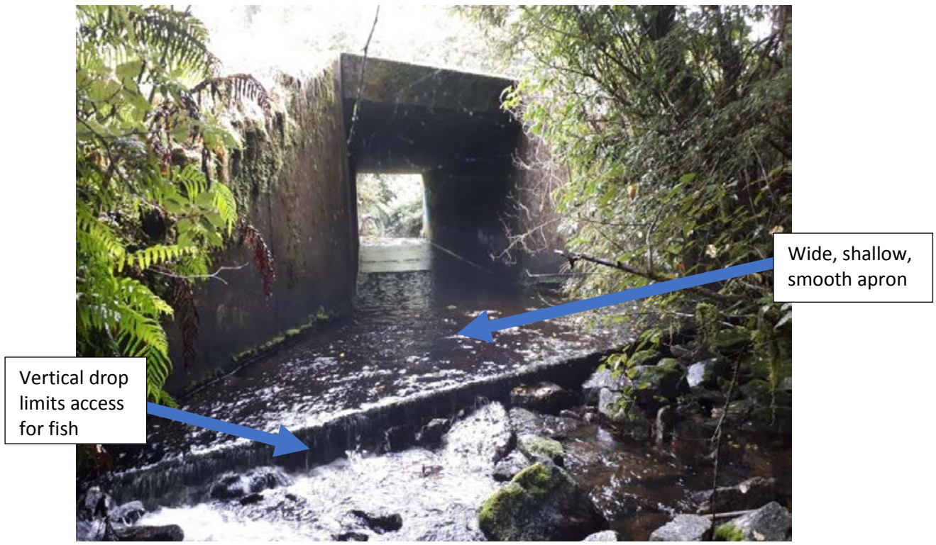
Figure E-17: Fish movements will be impeded by the fall at the downstream end of the apron and shallow water on the apron. Credit: Sam Ammon.
