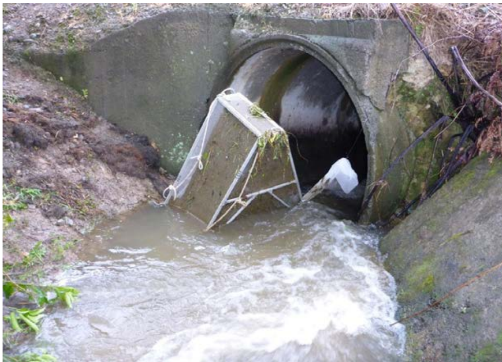
Figure I-10: Top trap during increasing flood waters at the conclusion of Trial 3.
