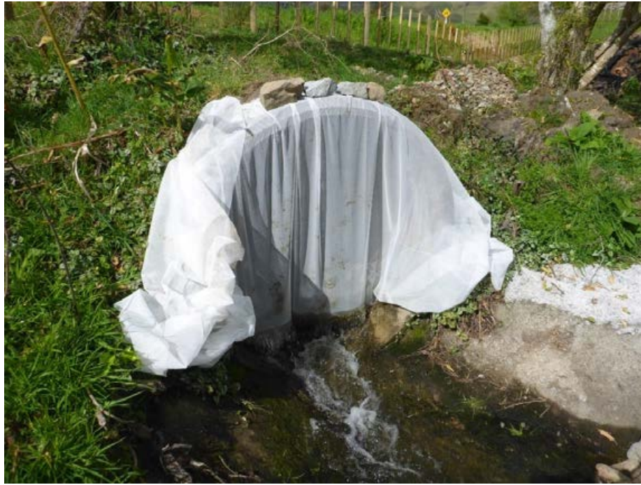
Figure I-8: Barrier net set upstream of the baffle at the culvert outlet.
