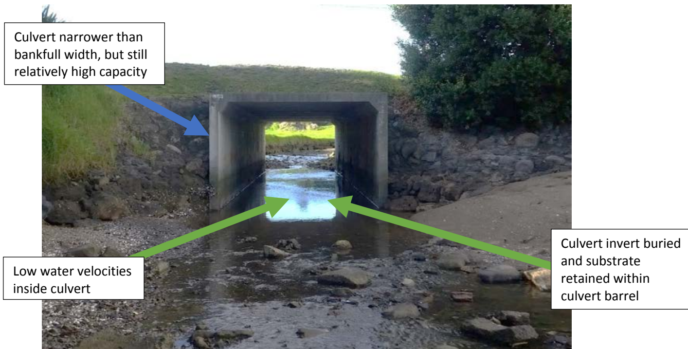
Figure E-22: Example of a culvert in a tidally influenced area. The culvert invert is embedded meaning that natural substrate is retained through the culvert. Culvert width relative to the stream bankfull width is lower than recommended, but because the culvert is in a tidal area, low water velocities will exist through the culvert during slack tide conditions. Credit: Bryn Quilter.
