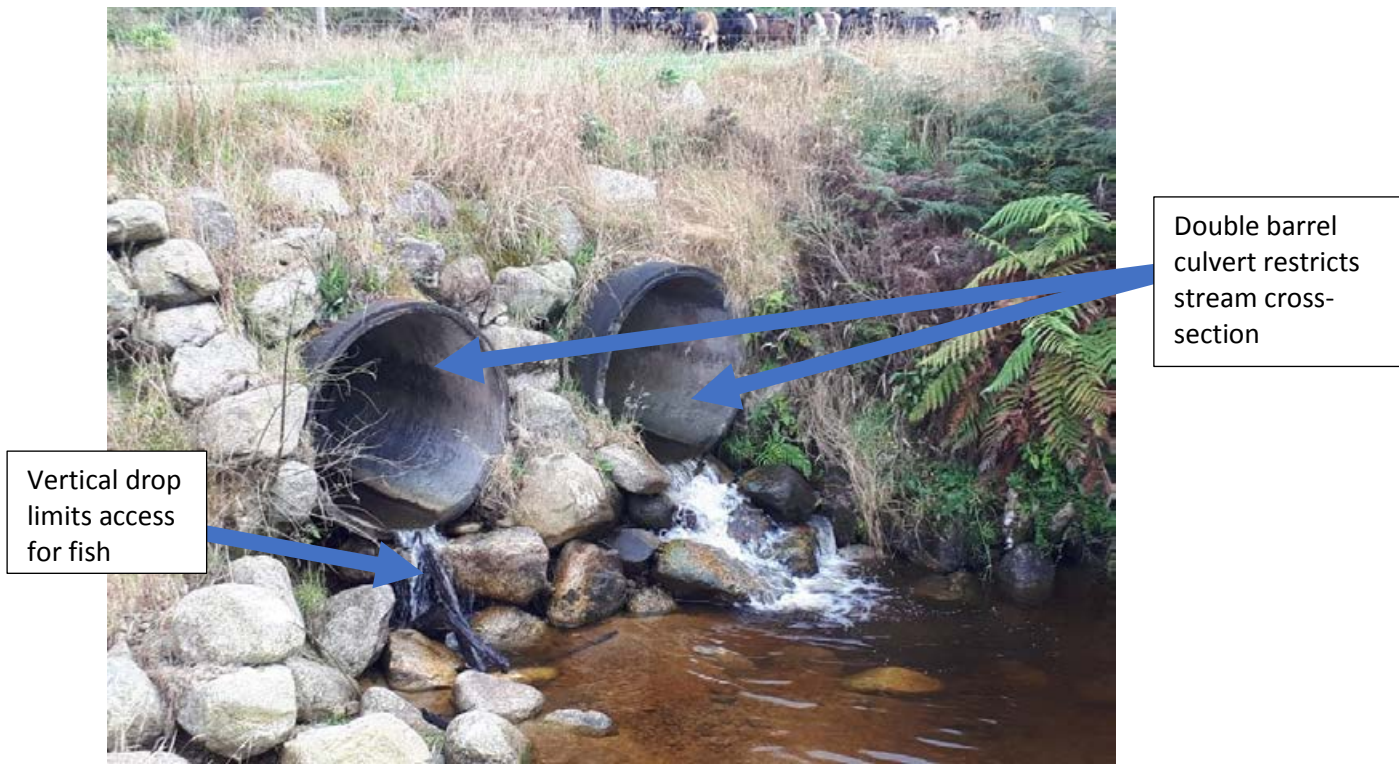
Figure E-16: A double barrel culvert where passage will be impeded by the fall height at the culvert outlet. Passage for climbing fish species may be possible over the rocks below the culvert in the right of the picture. Credit: Sam Ammon.
