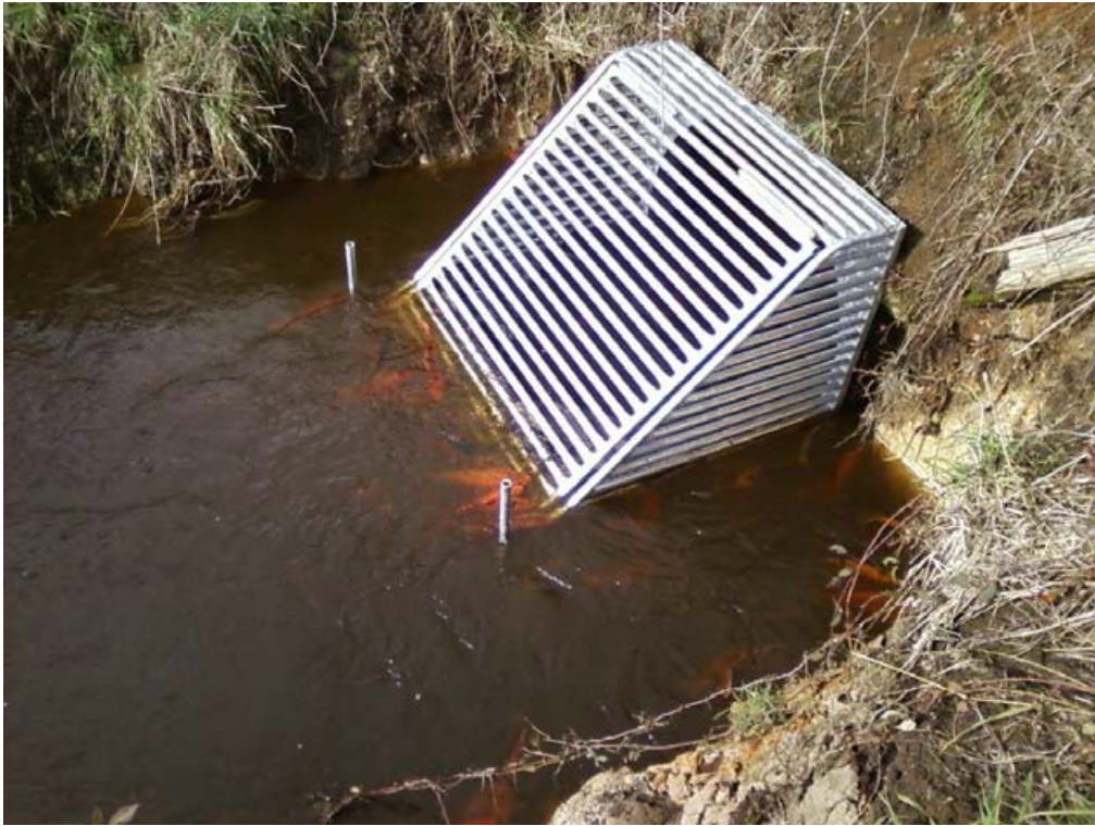
Figure 6-7: One-way gate fitted to Lake Ohinewai outlet drain, Waikato. The gate is designed to prevent adult koi carp from accessing the lake, while still providing small and other fish access to and from the lake. Credit: Adam Daniel.
