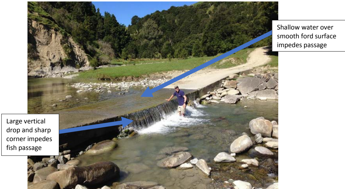
Figure E-21: The fall height on this ford on the Te Arai River is a significant impediment to the upstream passage of fish. Credit: Paul Franklin.
