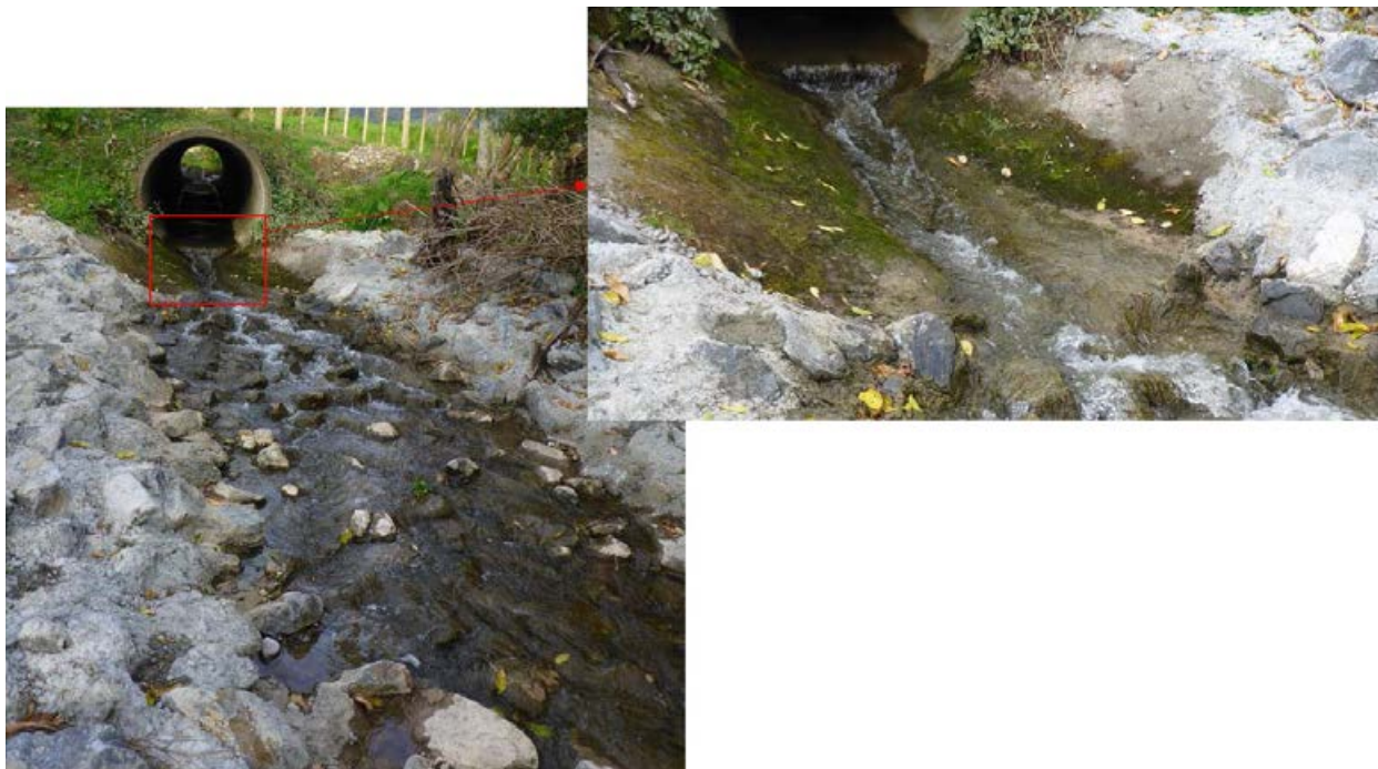
Figure I-1: Remediated culvert on Kara Stream, Upper Kingston Road. Inset shows the unmodified culvert apron.
