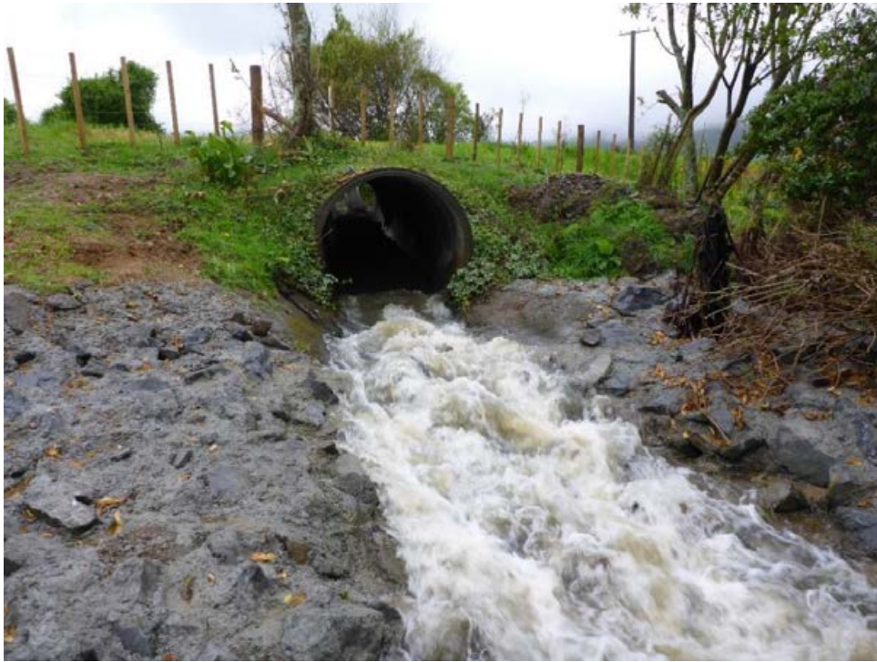
Figure I-11: Flow through the culvert and over the rock-ramp at the conclusion of Trial 3.
