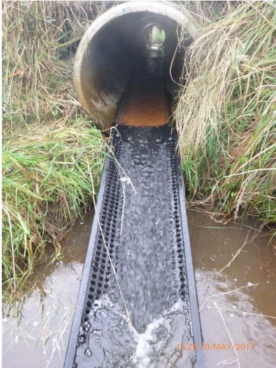
Figure 5-5: Example of an artificial fish ramp installed at a perched culvert in Southland. Note that a shallow wetted margin is maintained on both sides of the ramp. Photo: James Dare.
