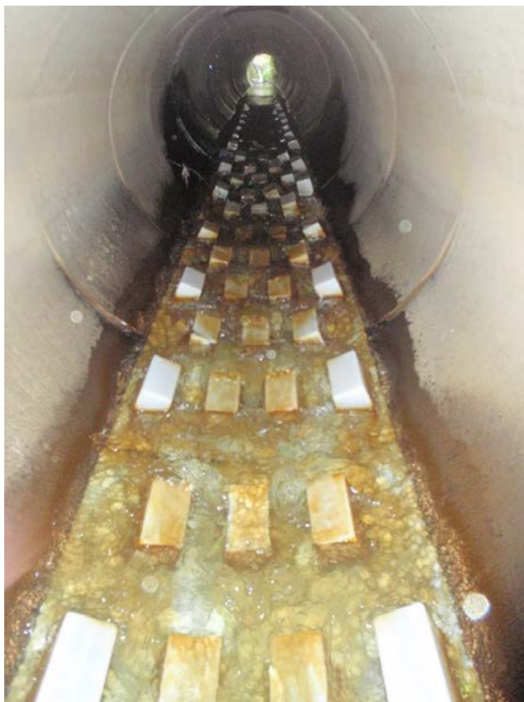
Figure 5-7: Spoiler baffle sheets installed inside a culvert.
