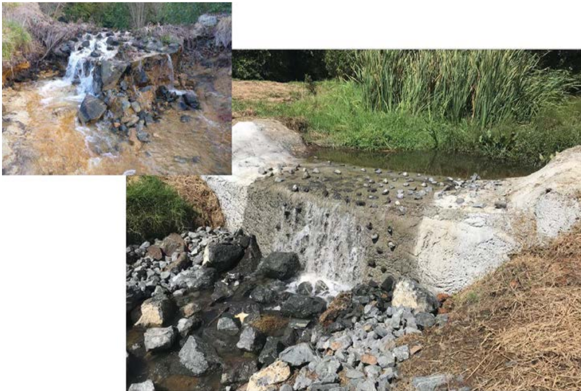
Figure 6-10: Baffled concrete weir in the lower reaches of Puketirini Stream, Waikato. A degraded weir (inset top left) was successfully preventing koi carp, goldfish, perch, rudd and gambusia from accessing upstream habitats whilst allowing the passage of banded and giant kōkopu, and shortfin and longfin eels. To continue protecting native fish populations the weir was remediated in 2018. Credit: Cindy Baker.
