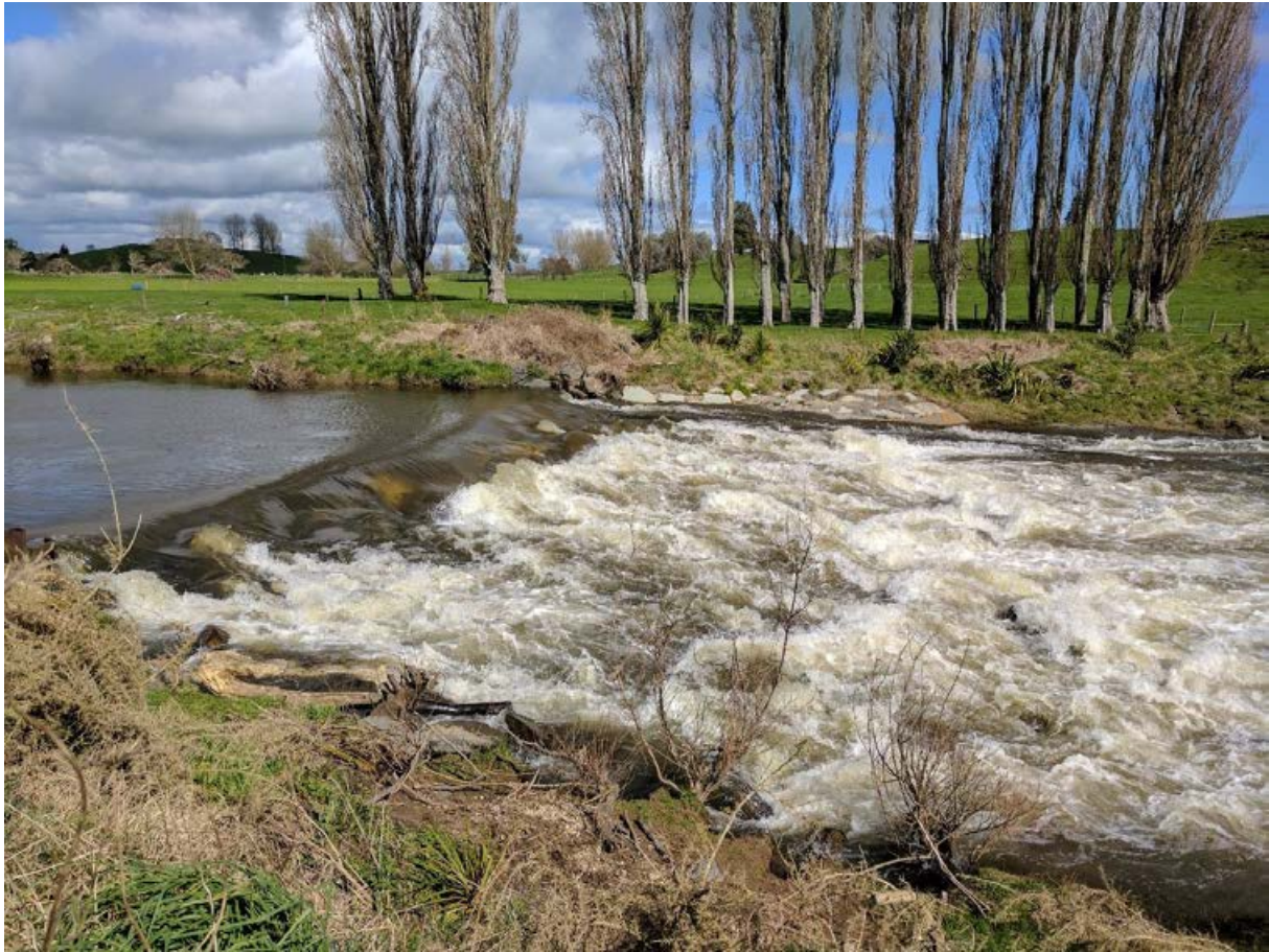
Figure 4-13: A rock-ramp style weir on the Waipa River at Otorohanga that also has a fish pass along the true left bank. The fish pass provides passage at low flows when the large rocks forming the downstream face of the weir are exposed and swimming species cannot surmount the weir. Credit: Eleanor Gee.
